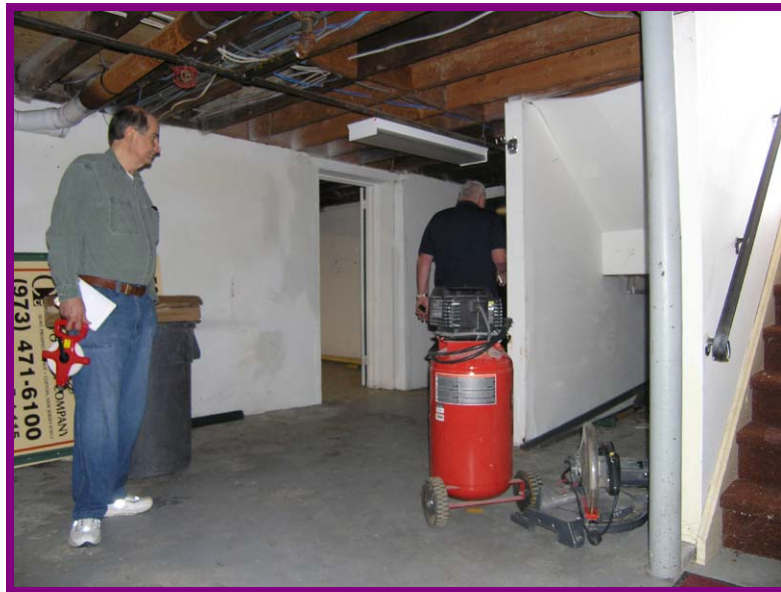
Inspecting the basement at Clifton
